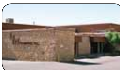
L&M Radiator, Inc. El Paso, Texas U.S.A.
