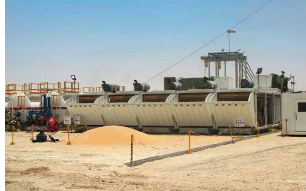
MESABI® radiators cooling Cat® 3512C P/N 115279. 1,476 horsepower good for 55c/131F ambient.
